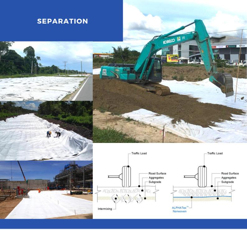
ALPHATex<sup>™</sup> nonwoven geotextiles has excellent mechanical properties catering to the load from cover material and irregular subgrades or stones.
