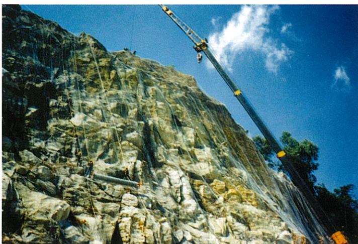
Erection of netting by means of crane, Penang – MALAYSIA
